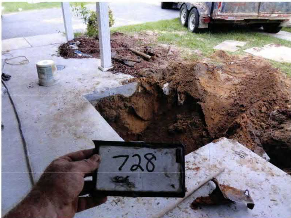
Picture 2: UST 728Bluebell excavation.
